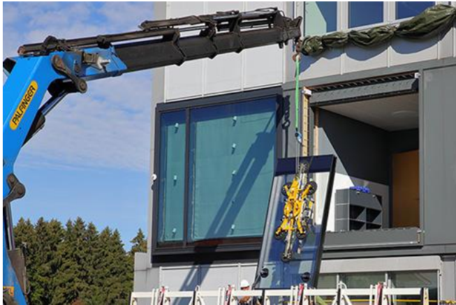
Installation of ISOshade elements from iconic skin GmbH in the VERU at Fraunhofer IBP © iconic skin GmbH
